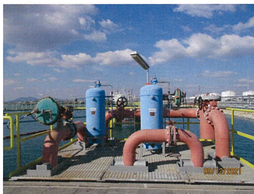
Fire Water Accumulator
